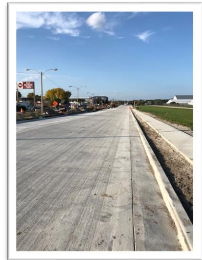
Photo of the newly reconstructed roadway, curb and sidewalk
