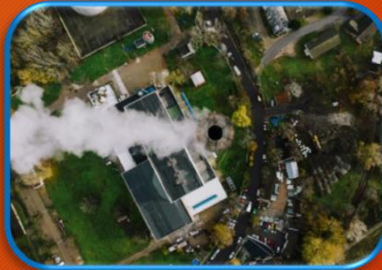
Smoke and Exhaust
