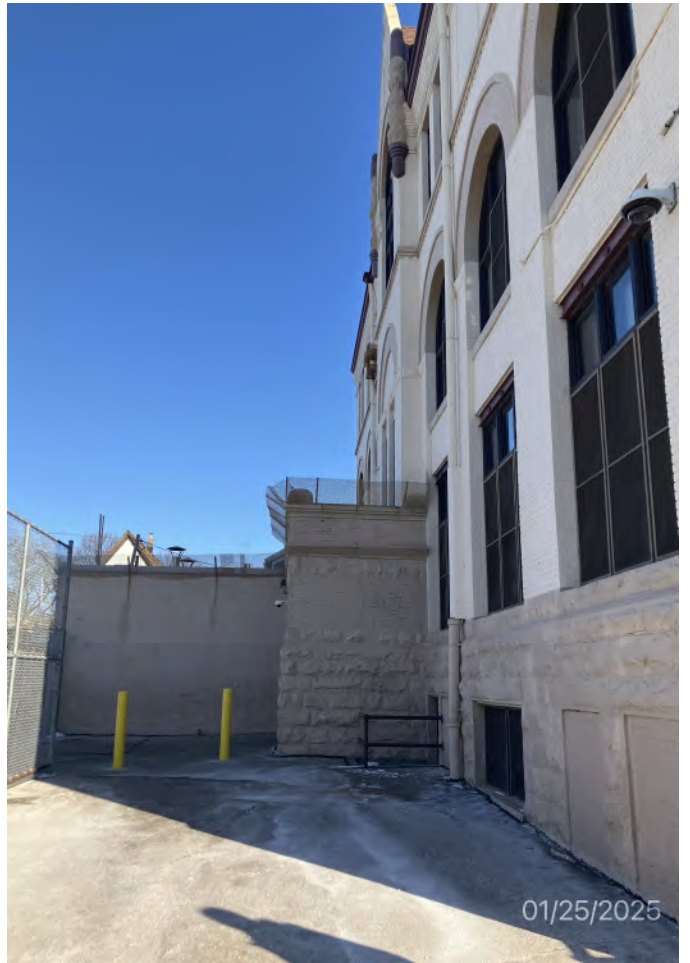
Exterior Side B
