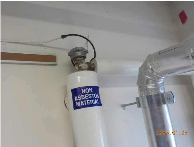
Rm 008A – East Wall D – deterioration (cracking)
