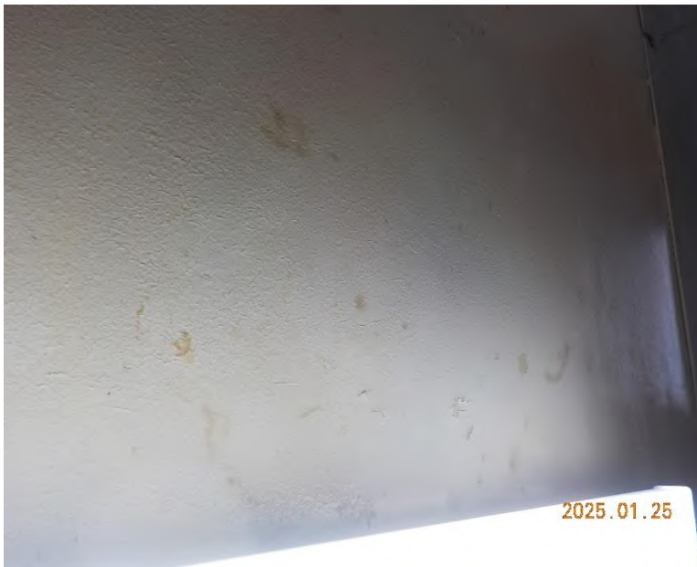
Girl's bathroom 009 - ceiling in sink area – deteriorated (peeling/chipped paint)
