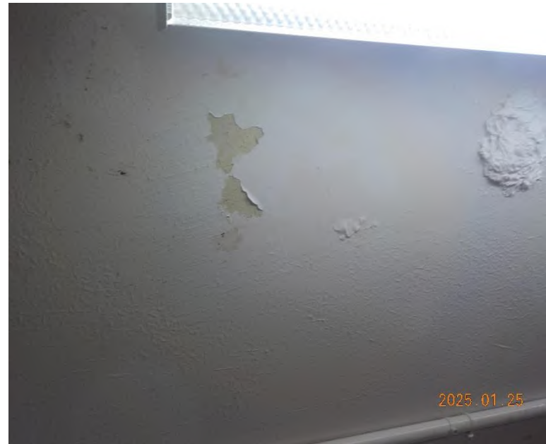
Girl's bathroom 009 - ceiling in sink area – deteriorated (peeling/chipped paint)
