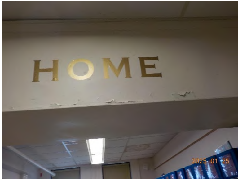
Rm 008A – HVAC duct (center of room) (peeling paint)
