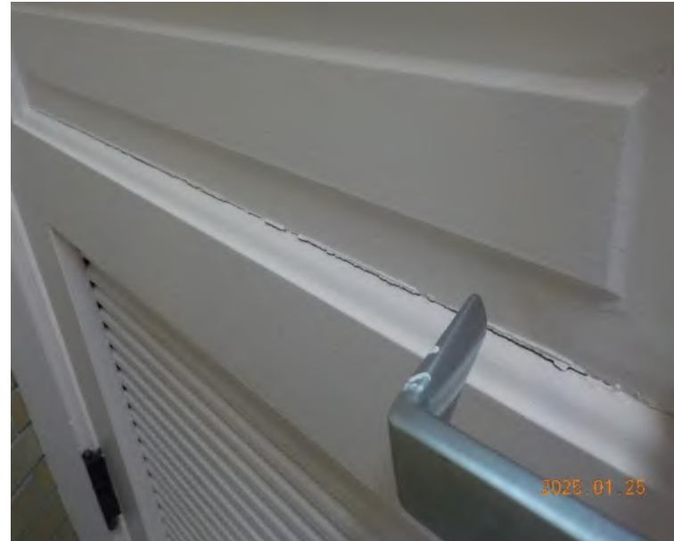
Girl's Bathroom 009 – both sides of right-side door from vestibule – (cracked/pickable paint deterioration)
