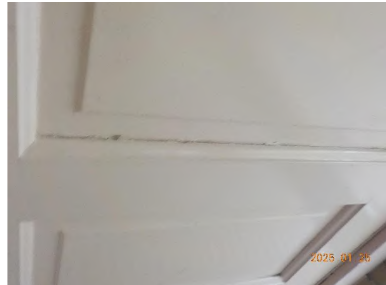
Room 002A – door-jamb & door (cracked/pickable paint)
