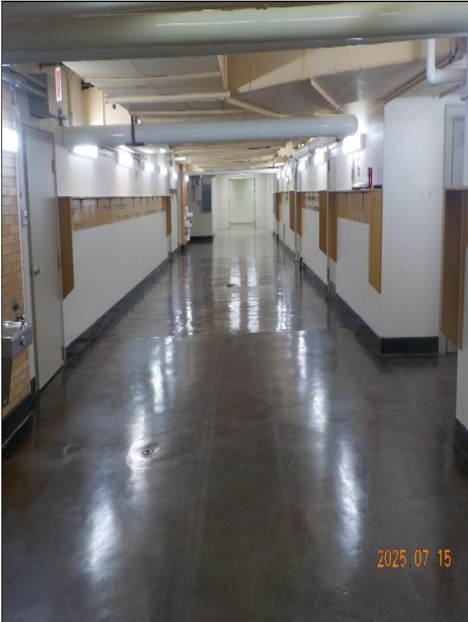
Corr. G-1 view south to north
