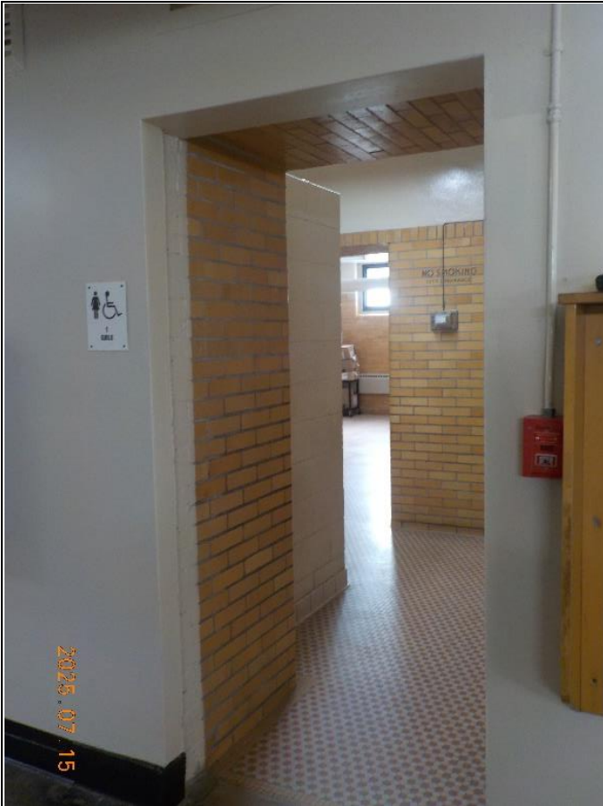
Corr. G-1 outside Girls' Toilet (001)
