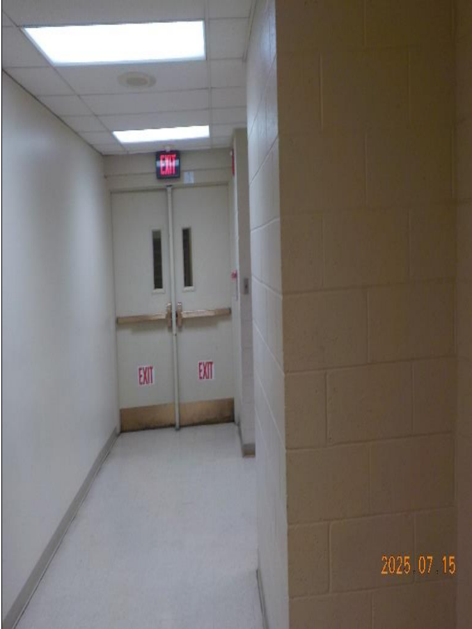
Corr. G-3 view west to east
