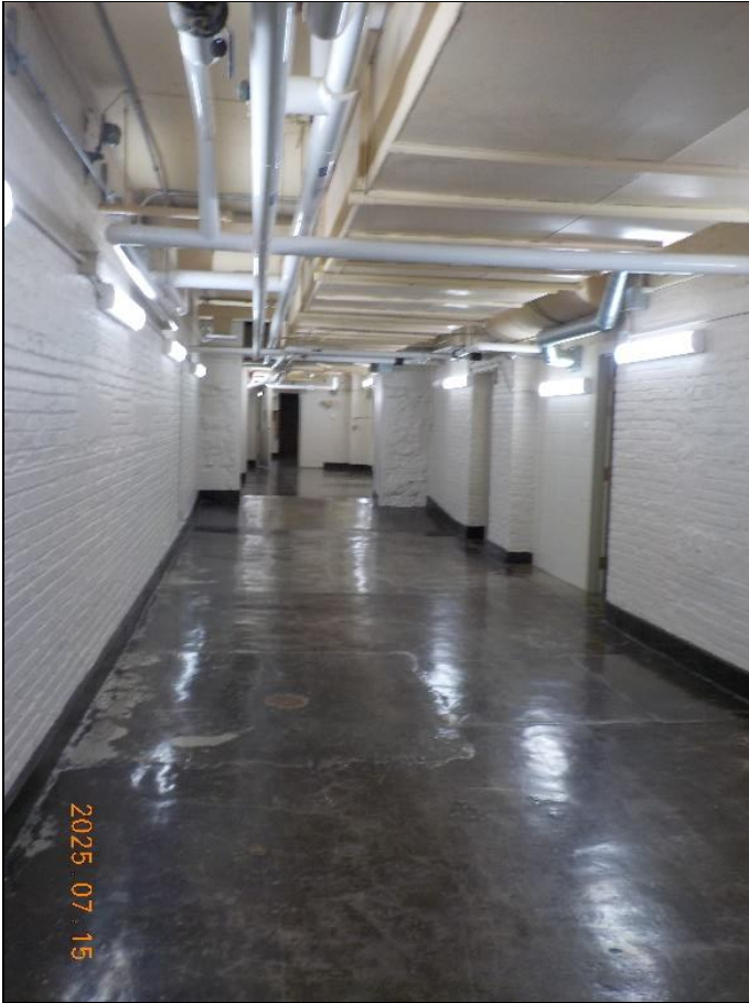
Corr. G-2 view west to east
