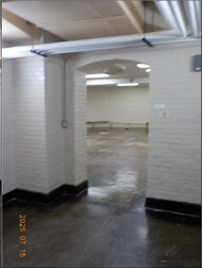
Corr. G-2 view into Room 012
