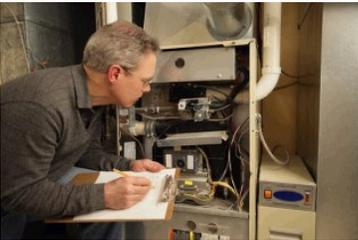
New, high-efficiency gas furnaces and boilers save significant amounts of energy in heating your home. Older types of gas furnaces and boilers allow more than 25% of the heat from gas combustion to exit through the flue exhaust stack or chimney. ENERGY STAR® labeled furnaces and boilers are designed to allow less than 10% of the heat to escape. More than 90% of the heat is used to warm your home. The advanced features of these new furnaces and boilers reduce energy waste and save you money.
