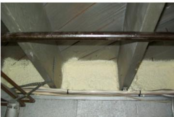
Rim joist insulation prevents conductive heat transfer through your home's floor system into a conditioned basement. In terms of comfort, adding rim joist insulation will make a noticeable difference in how warm your floor feels, especially in homes with wood or tile floors and for those who prefer not to wear shoes at home. At a minimum, the outer perimeter of the floor system, the rim joist, should be insulated to prevent heat transfer between the floor space and the outside.
