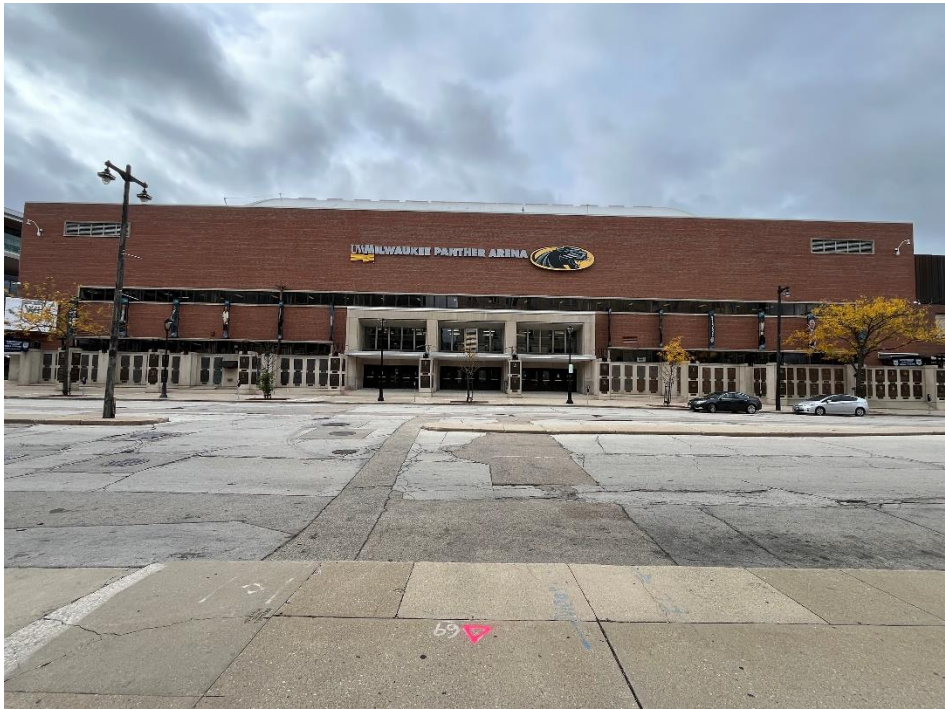
Figure 22 East façade of the Arena, 2025.
