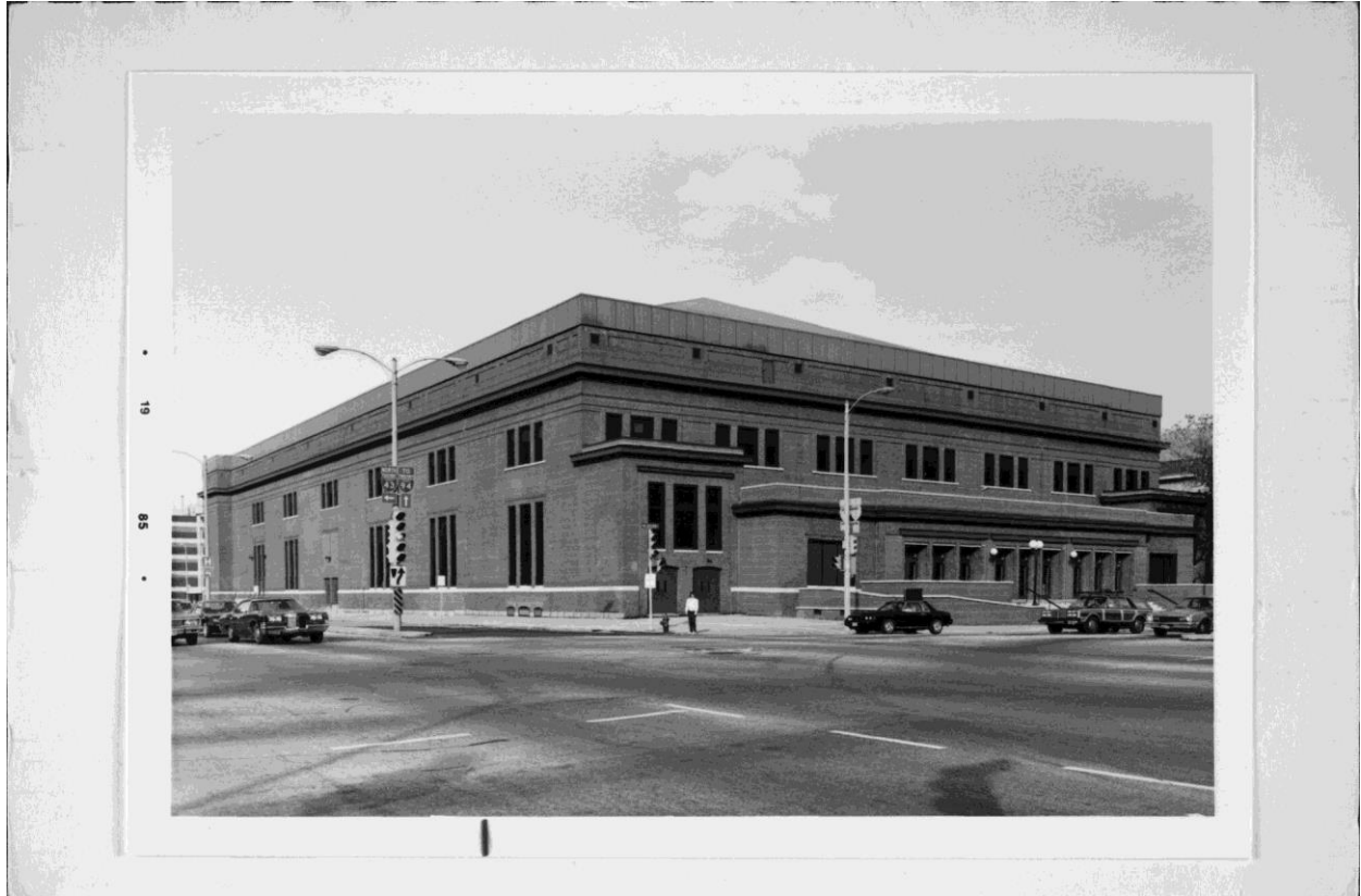
Figure 9 Auditorium, 1985. Wisconsin Architecture and History Inventory #73319.
