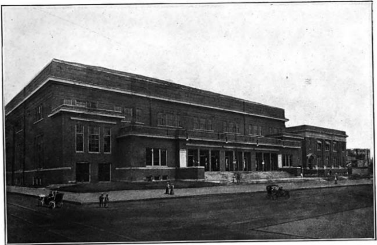
ENTRANCE ON CEDAR STREET.
