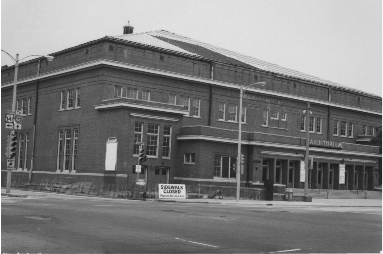
Figure 8 Auditorium, 1975. Wisconsin Architecture and History Inventory #73319.
