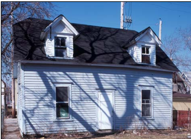
The carriage barn behind the Kren building is one of the better-preserved late 19 th century structures of its kind on the near north side.
