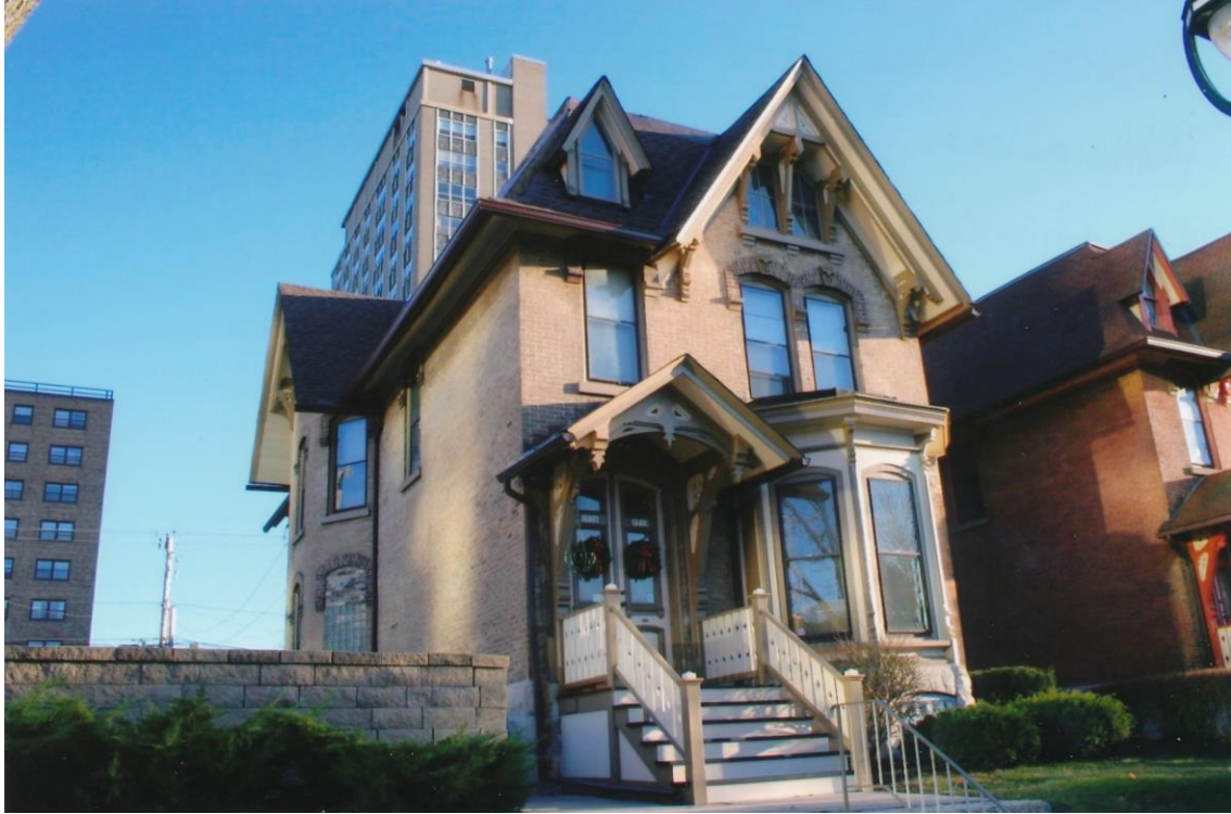
Figure 14. Justus & Margaret Vallat House, 1714-1716 N. Farwell Avenue. Wisconsin Architecture and History Inventory, Record # 106615. Photo taken 2010.
