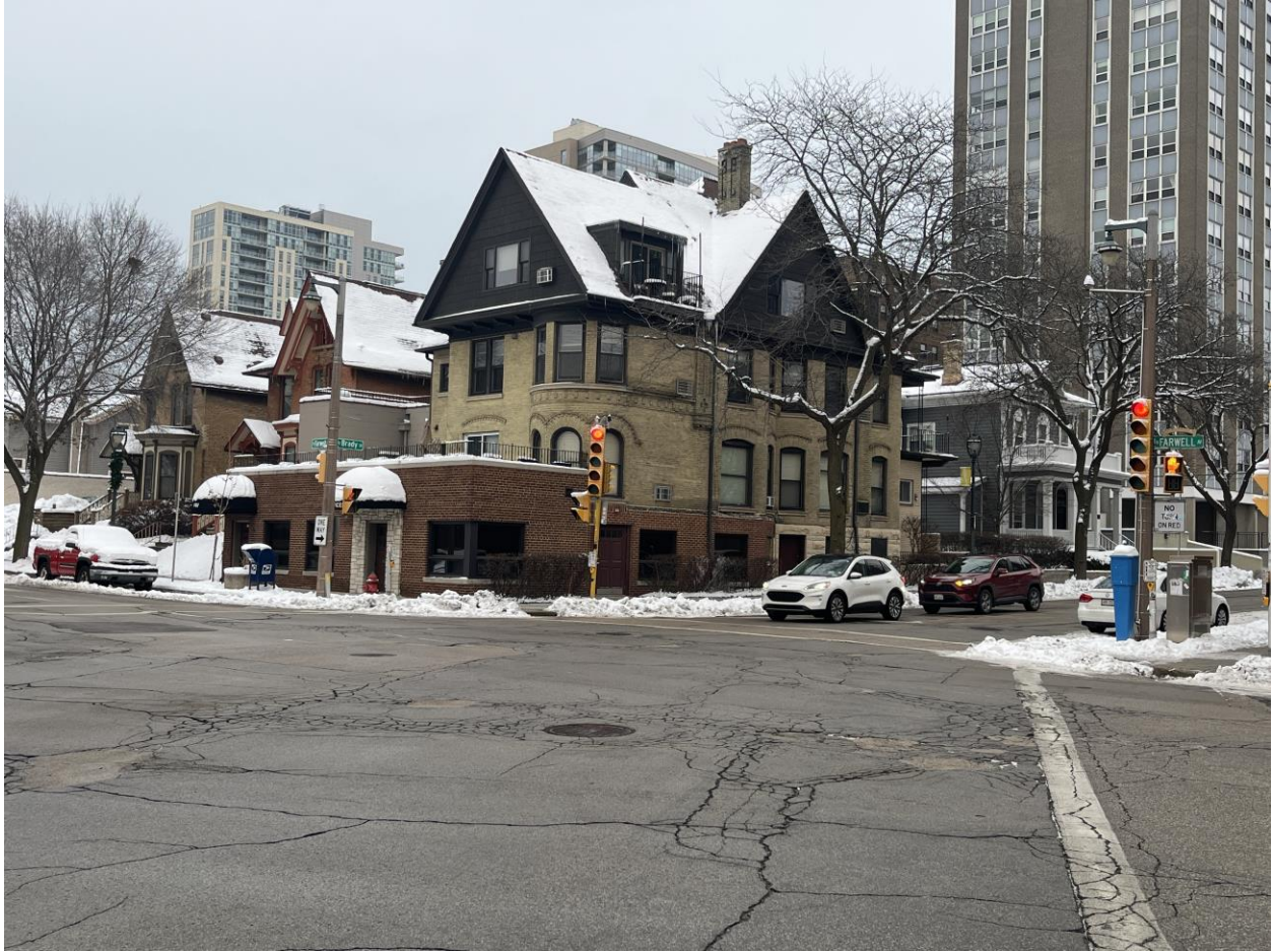
Figure 16. Brady & Farwell Historic District, photo taken 2025.
