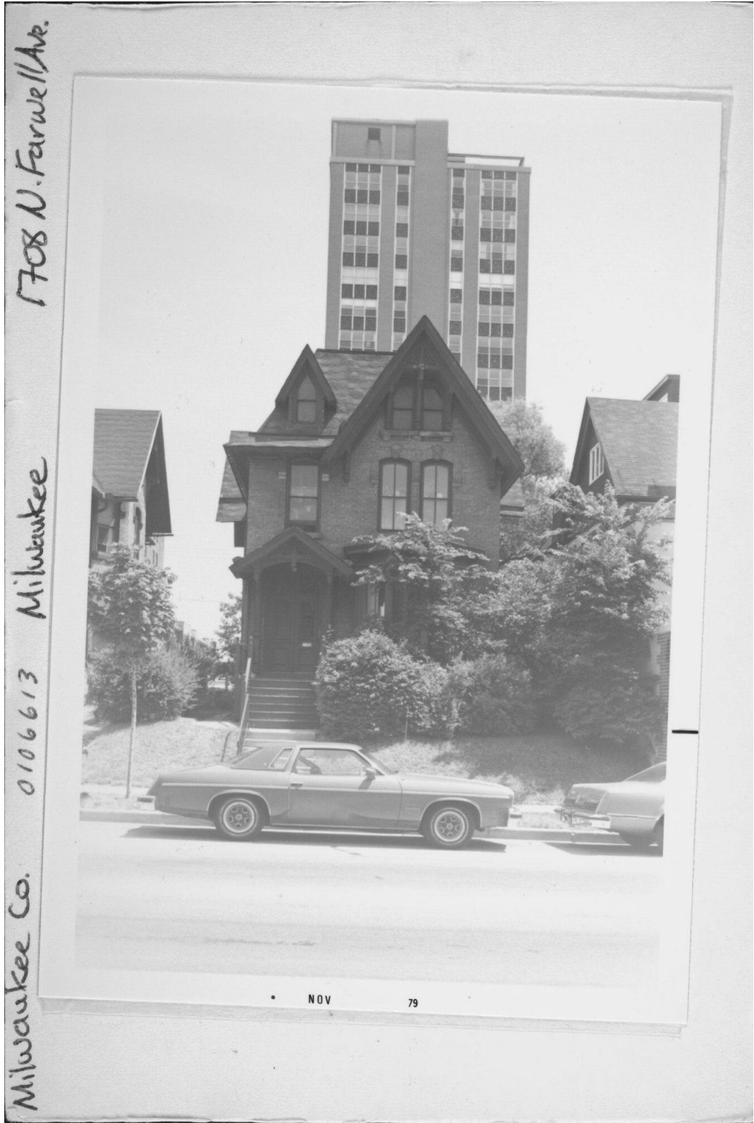
Figure 8. Justus & Margaret Vallat House, 1708 N. Farwell Avenue. Wisconsin Architecture and History Inventory, Record # 106613. Photo taken 1979.
