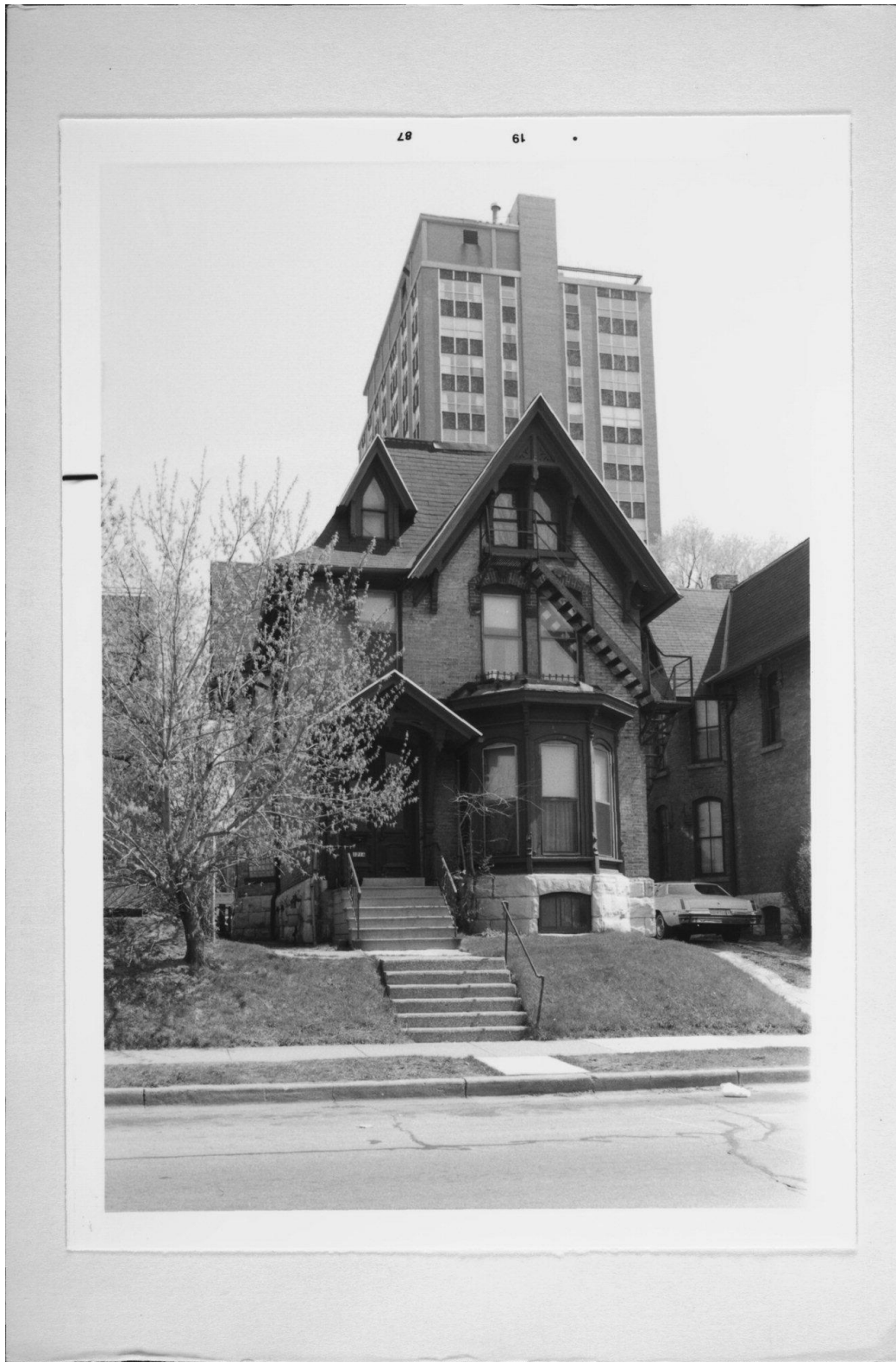
Figure 13. Justus & Margaret Vallat House, 1714-1716 N. Farwell Avenue. Wisconsin Architecture and History Inventory, Record # 106615. Photo taken 1987.
