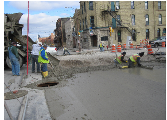
Crews installing concrete at South 2nd Street at Virginia
