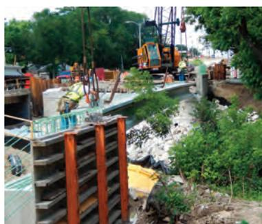
Girders were lowered into place as part of the reconstruction of the bridge over the Menomonee River. Thanks to the coordinated efforts of the contractor, Lunda Construction, the City of Milwaukee, the City of Wauwatosa and the Wisconsin Department of Transportation, traffic flow was uninterrupted during the girder installation.
