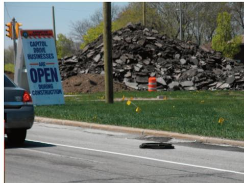
The general contractor Stark Electric, along with several sub contractors, has started removing old pavement, milling, grinding and grading. The removed pavement is piled up on the north side of the project to be used later as fill for the roadway (photo).
