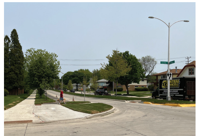
Curb extension at Griffen & Howard
