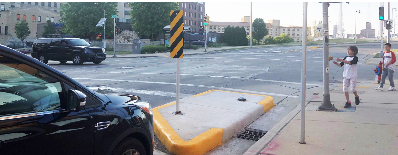
Pinned-on Curb Extension on S. 6th Street
