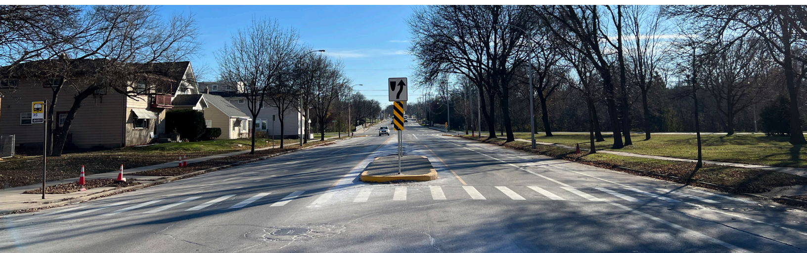
Traffic Island, Full Concrete
