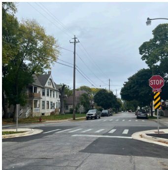
Curb Extension, Full Concrete
