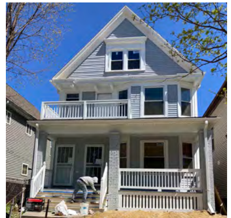
Finishing touches at North 29th Street.
