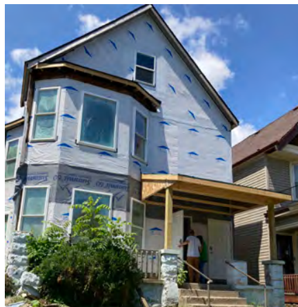
Home rehab in progress.
