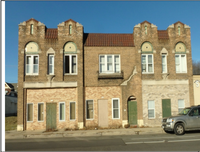
5008-14 West Center Street
