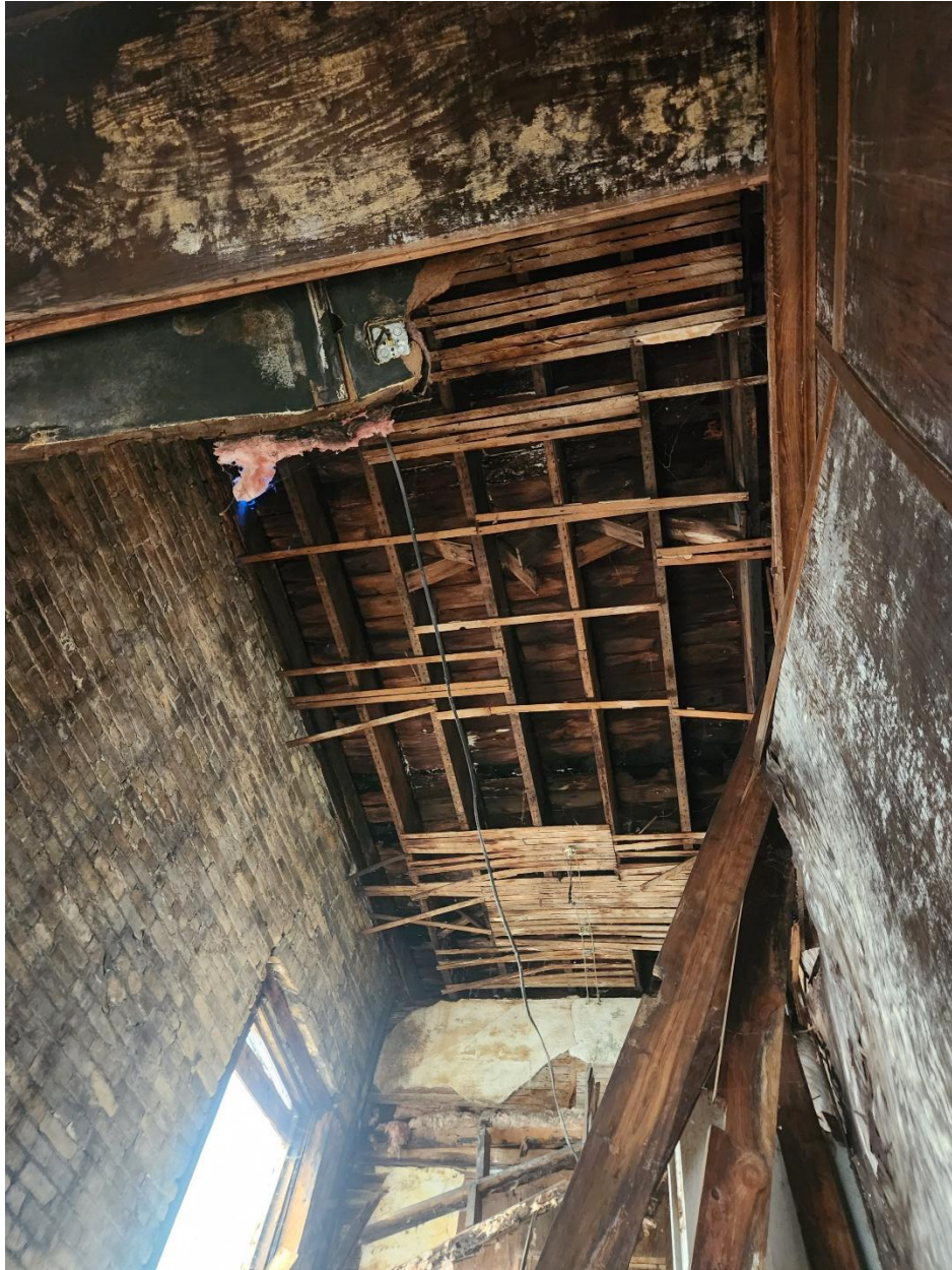
3 rd Floor Roof Underside
