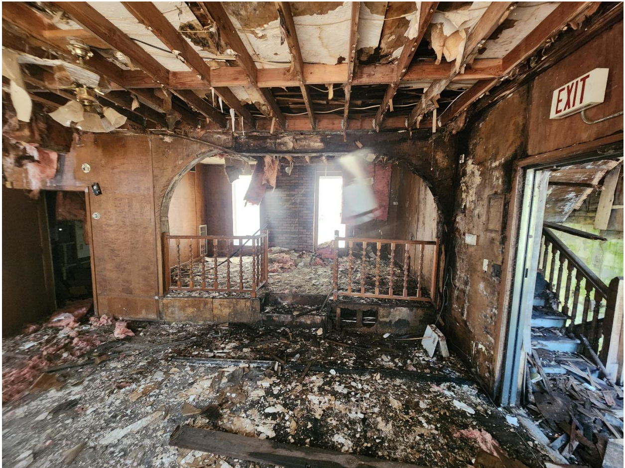
2 nd Floor East Archway
