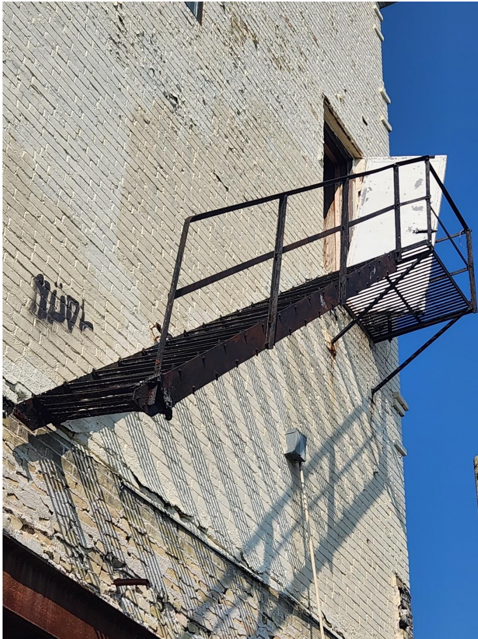
3 rd Floor South Fire Escape
