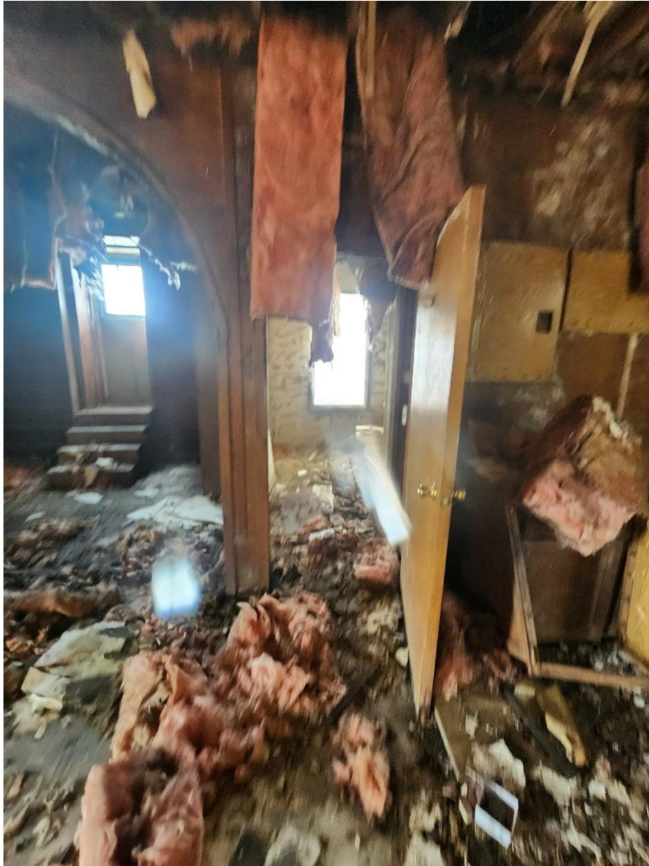
2 nd Floor Bathroom
