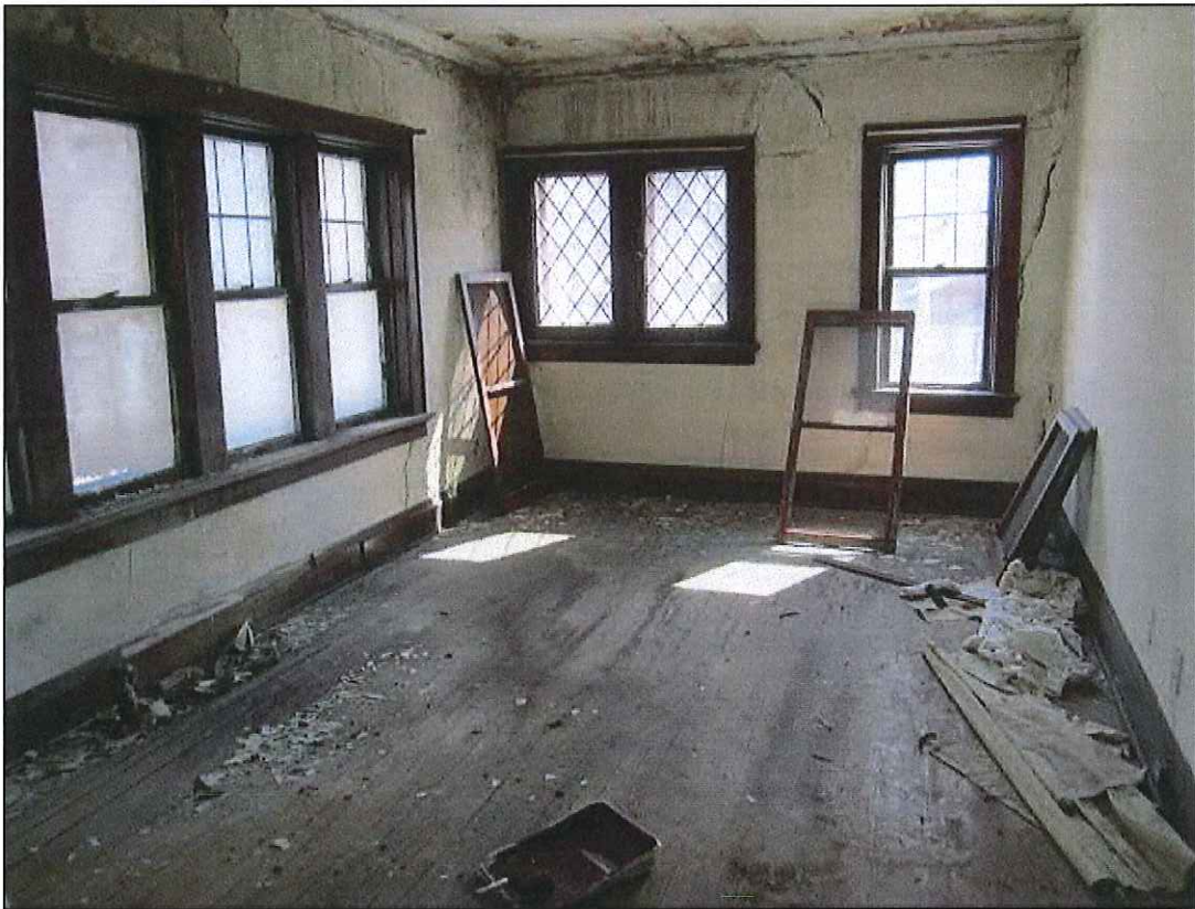
View of an apartment on the second floor of the building.
