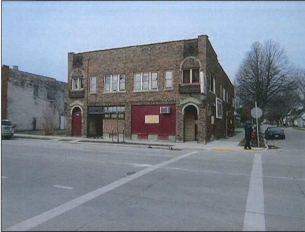
View of project site, looking west from N. Port Washington Avenue.
