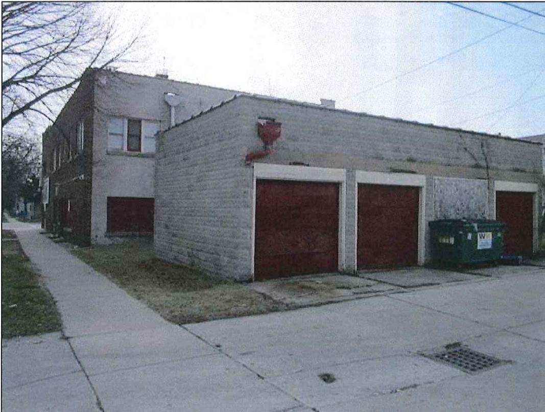
View of the project site, looking east from the alley.
