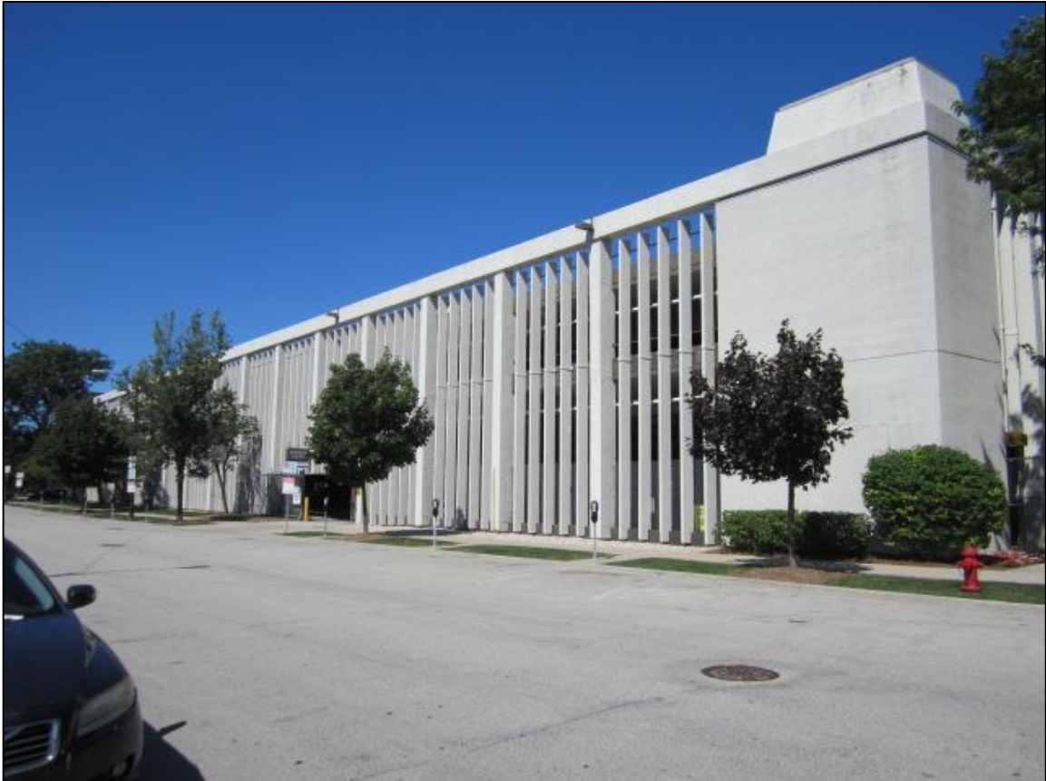
View of project site facing northeast.
