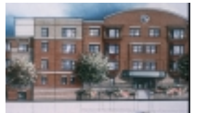
The Library Hill residential /mixed-use development is located between 7th and 8th street is currently under construction.
