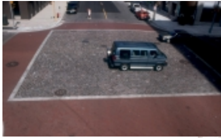
Enhanced intersection and defined crosswalk
