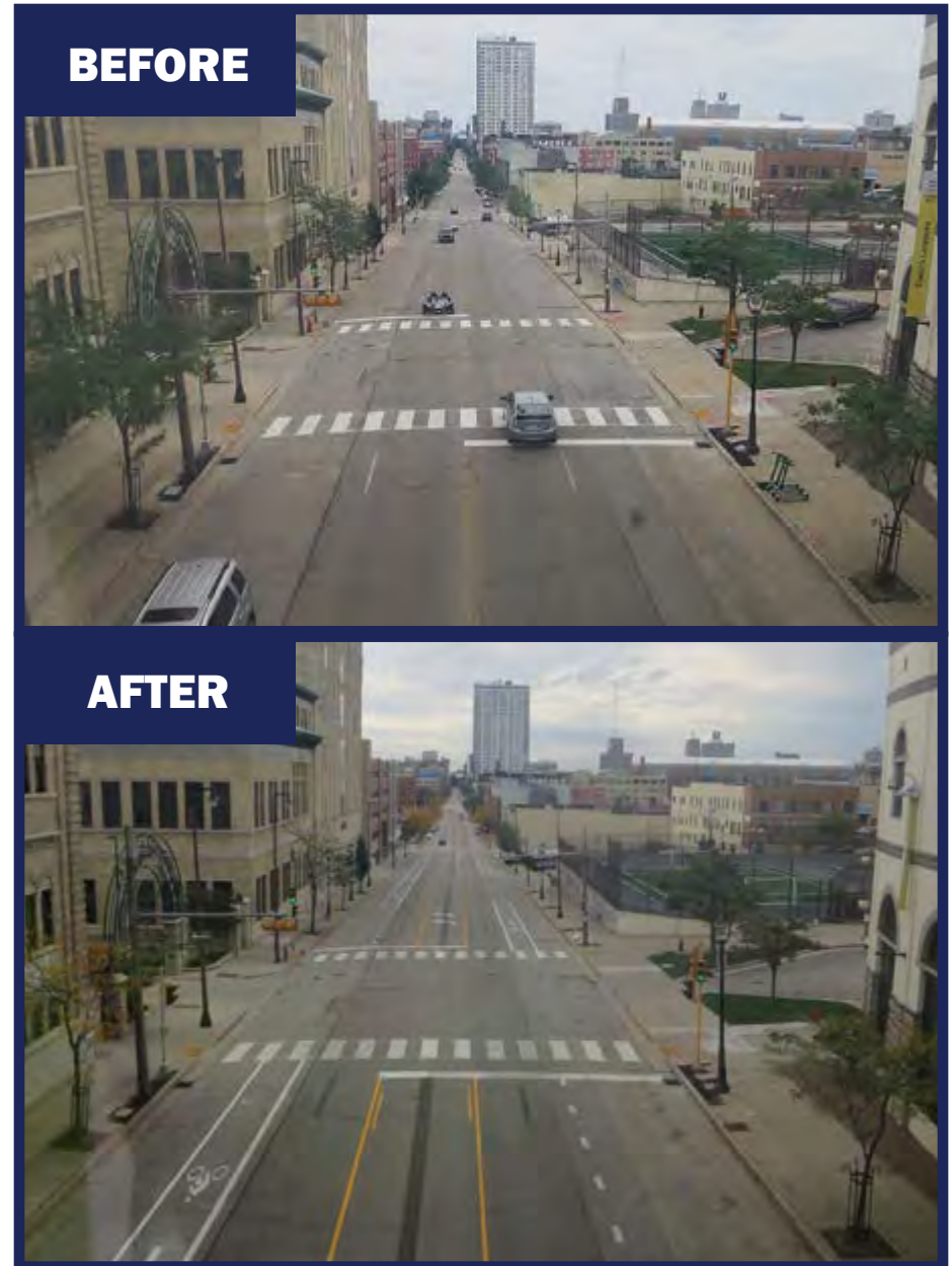
Before and after photos of a road diet on N. Doctor Martin Luther King Jr. Dr.
