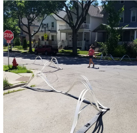
Figure 2: Wave delineators used as temporary curb extensions
