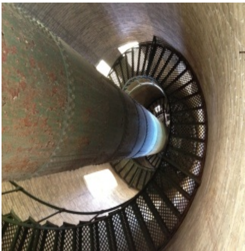
As visitors stepped into the 14-foot-wide North Point Tower they stood face-to-face with the 135-foot-tall iron standpipe that once was part of a steam engine system that pumped Lake Michigan water for fire suppression and drinking. Visitors saw a display of historical photos dating back to the 1870s, when cows grazed outside the tower on what was then farmland north of downtown Milwaukee.
