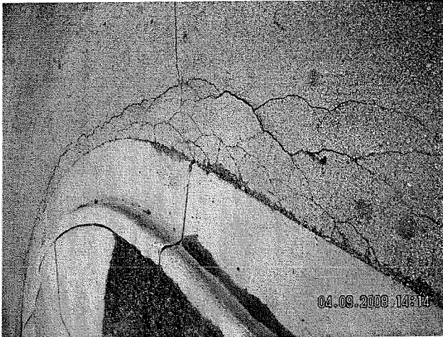
Photo of Alligator Cracking at the edge of pavement
