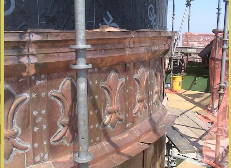
Raise copper panels on the south tower drum.
