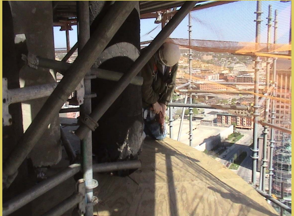
Installation of new wood decks on the lantern of the south tower.
