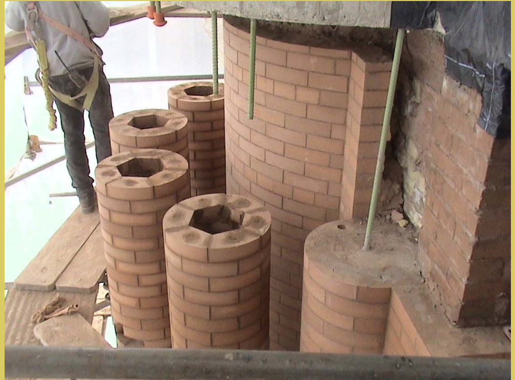
Continued brick work on the south tower.
