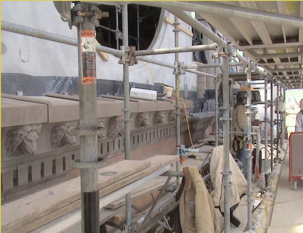
Boarder of small lion heads installed on clock precast.
