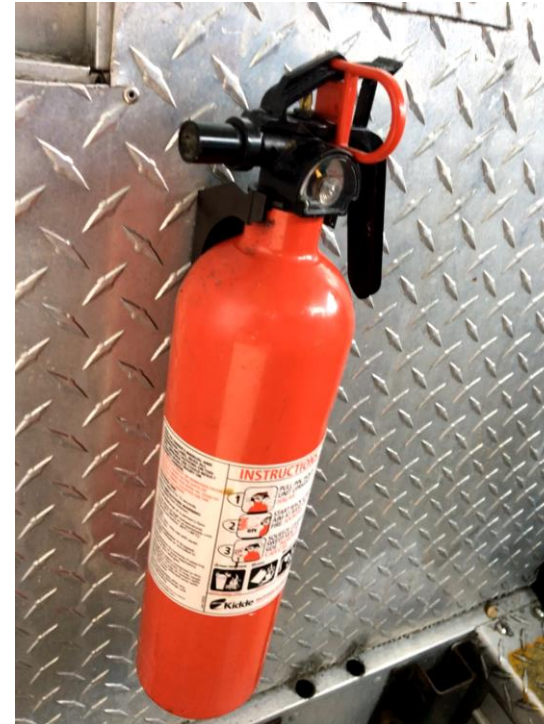
ABC fire extinguisher for all other types of mobiles that use fuels
