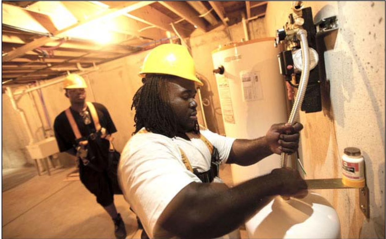
Denton Naylor connects a fluid pump to an expansion tank while installing a hot water solar system in the basement of a home under construction Thursday in Milwaukee. (Staff photos by Kevin Harnack)
