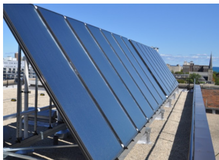
Solar thermal install at MSOE residence hall
