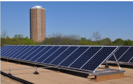
New solar install at Riverside High School
