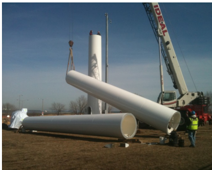
Wisconsin-made tower being craned into place
