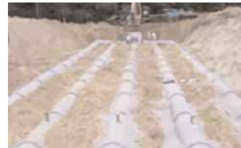
Earth pipe/concrete pipe system
