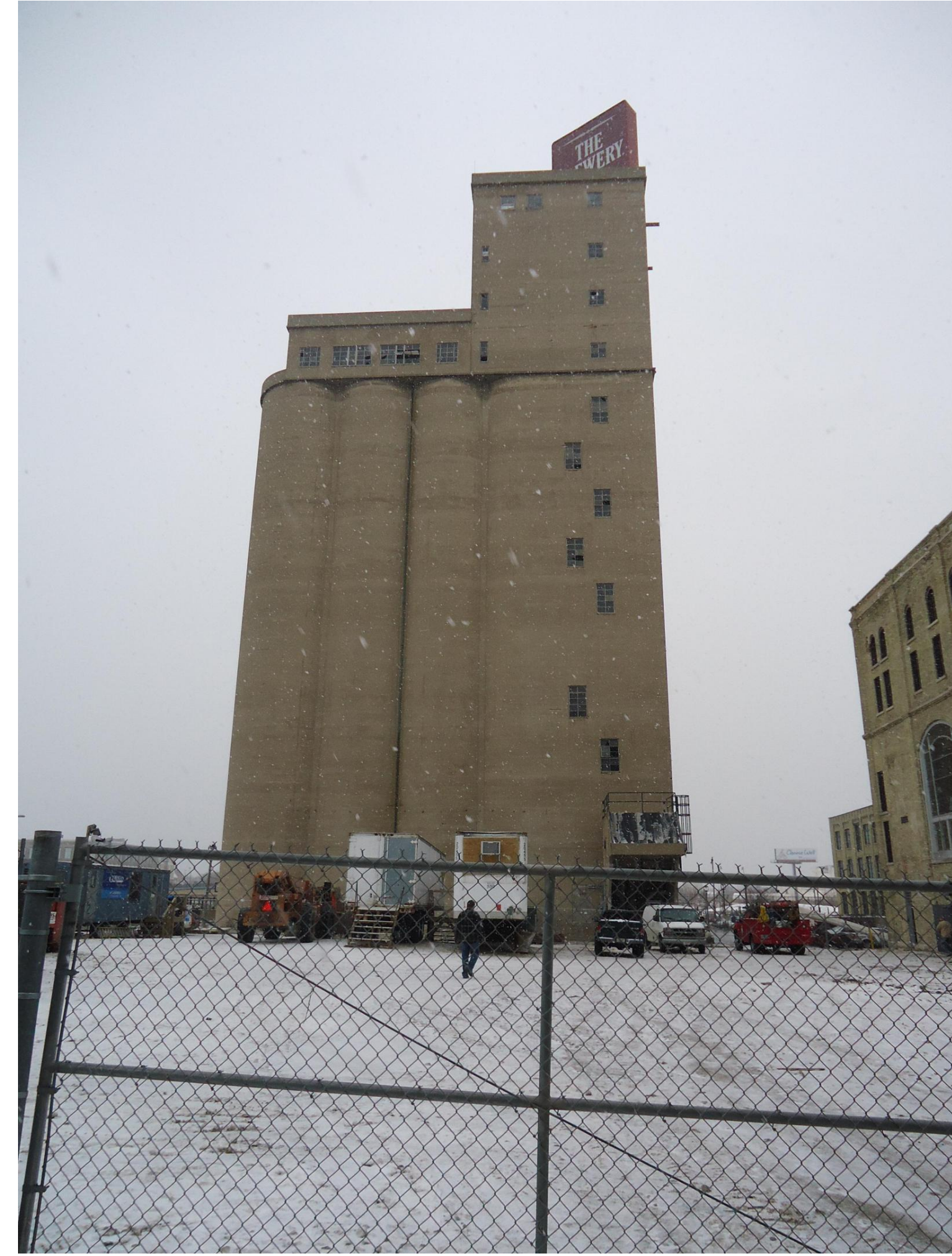
CONCRETE GRAIN SILOS TO THE NORTH
