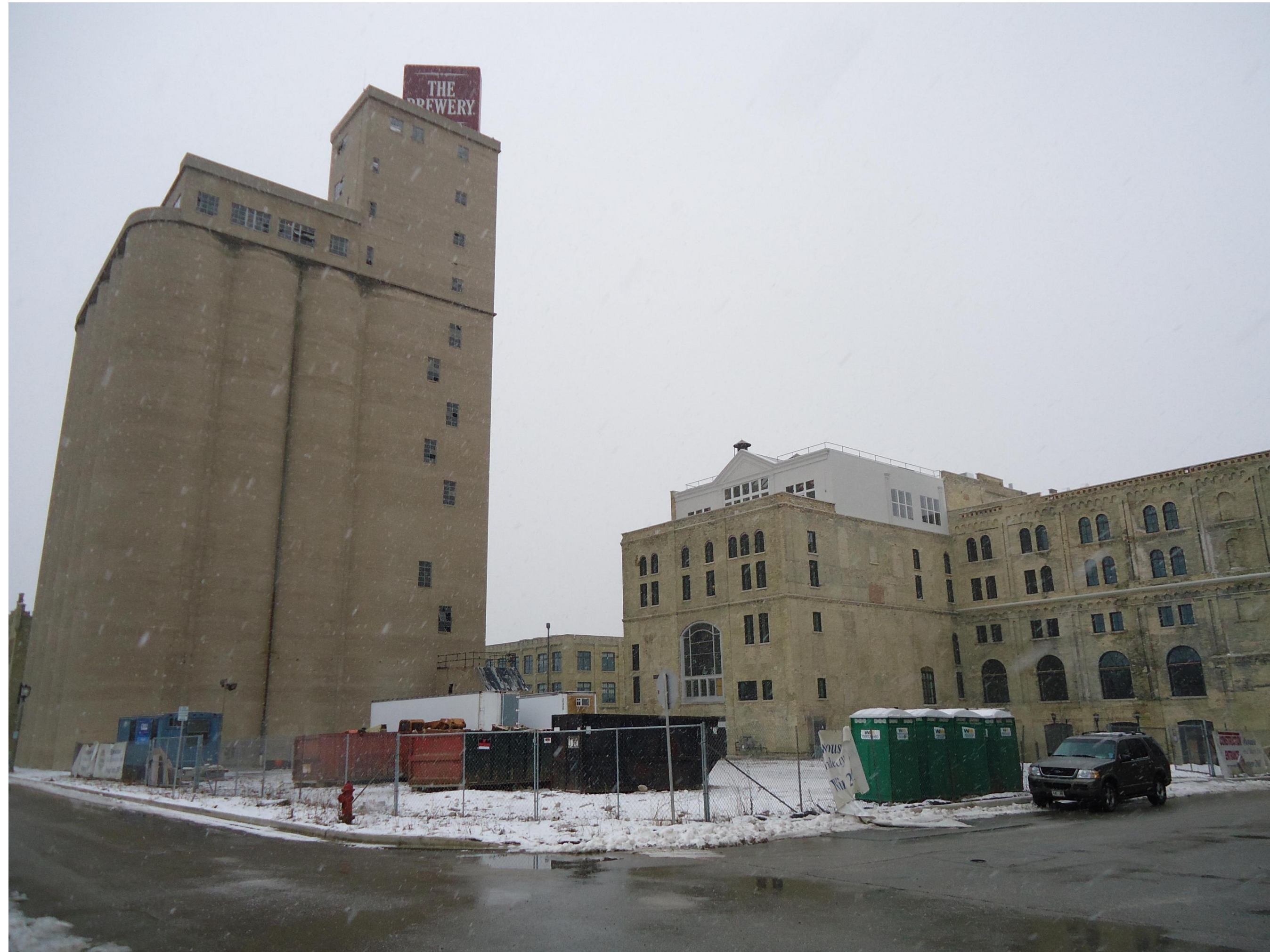
VIEW OF THE PROJECT SITE - LOOKING NORTH EAST
