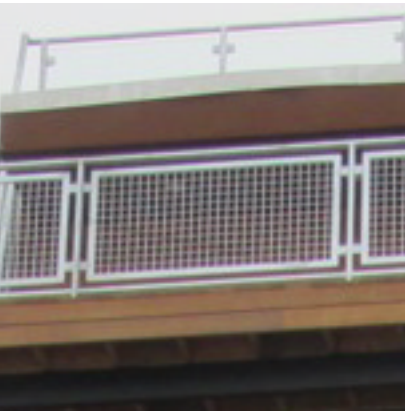
WIRE MESH IN-FILL
