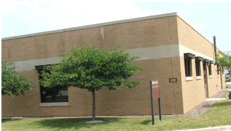
Exhibit III-8: Building 222 Aircraft Maintenance/Flightline Facility
