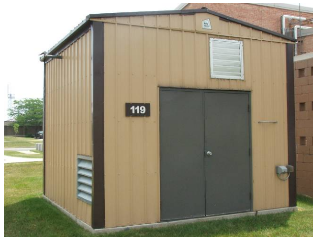
Exhibit III-14: Building 119 Emergency Generator for Building 107
