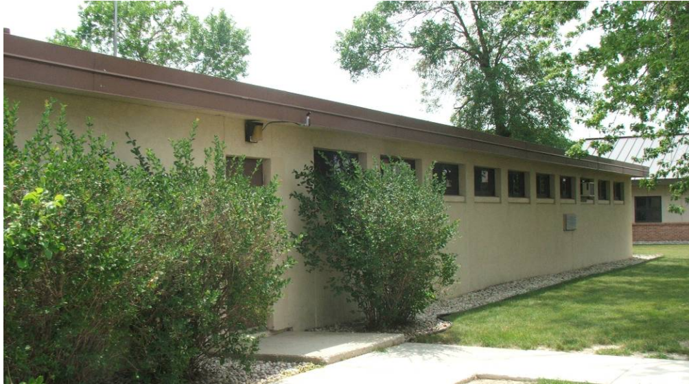
Exhibit III-12: Building 110 Billeting/Fitness Center
