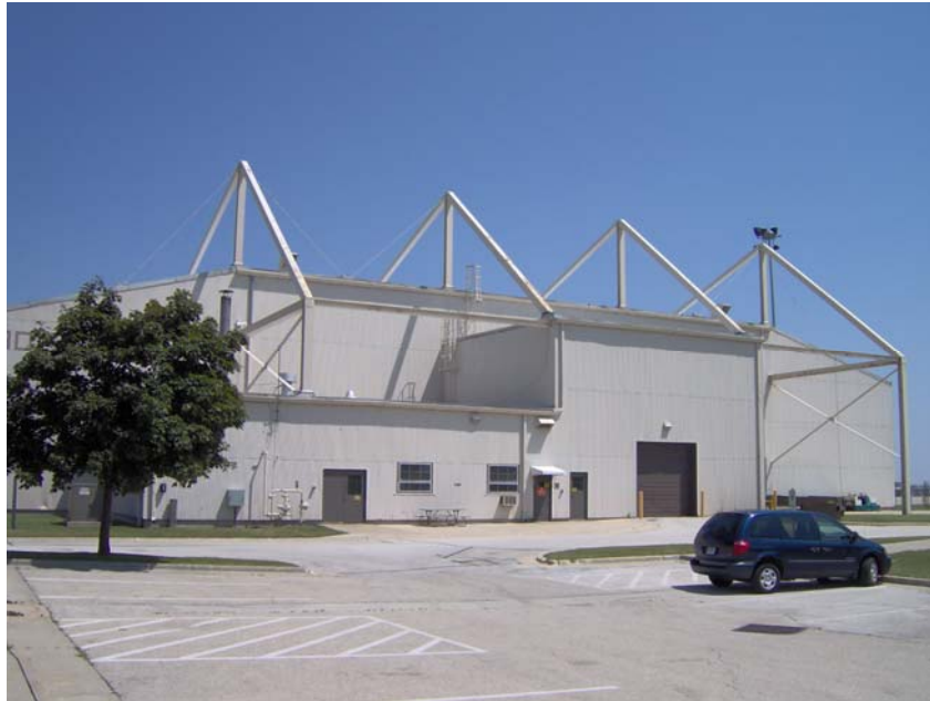
Exhibit III-5: Building 302 Fuel Systems Maintenance Dock
