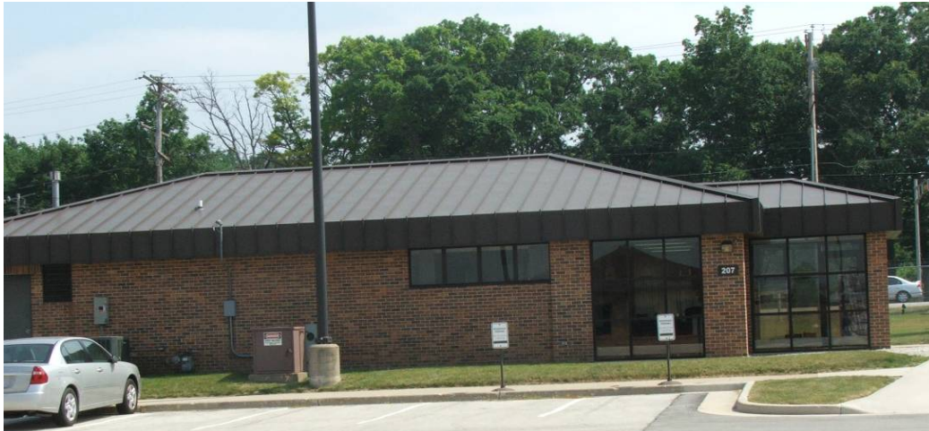
Exhibit III-3: Building 207 Recruiting Office at Front Gate
