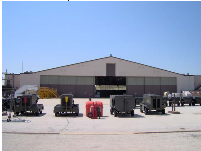
Exhibit III-6: Building 217 Maintenance Hangar
