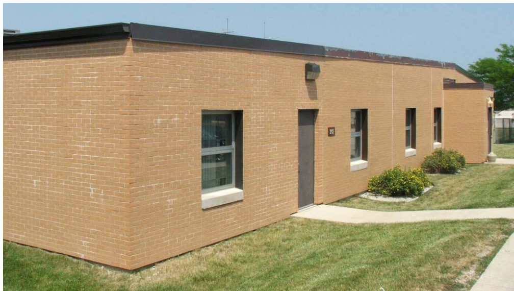
Exhibit III-11: Building 212 Fire Station
