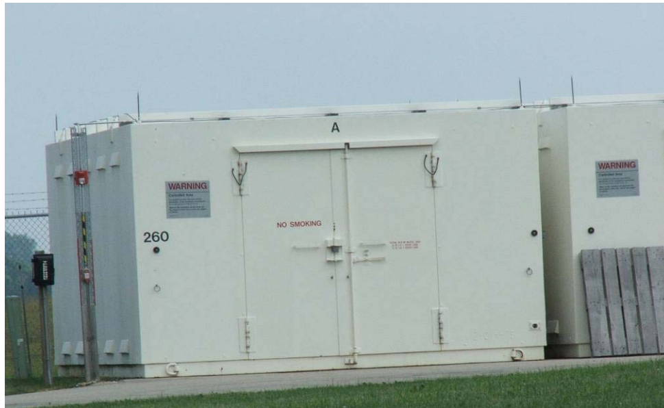
Exhibit III-15: Building 260A Munitions Storage
